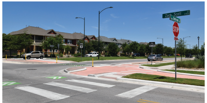
Protected intersection at Zach Scott St. and Berkman Dr.
