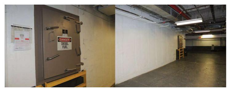
Figure 5-5. Dry floodproofed fuel tank enclosure in basement of a high-rise building
