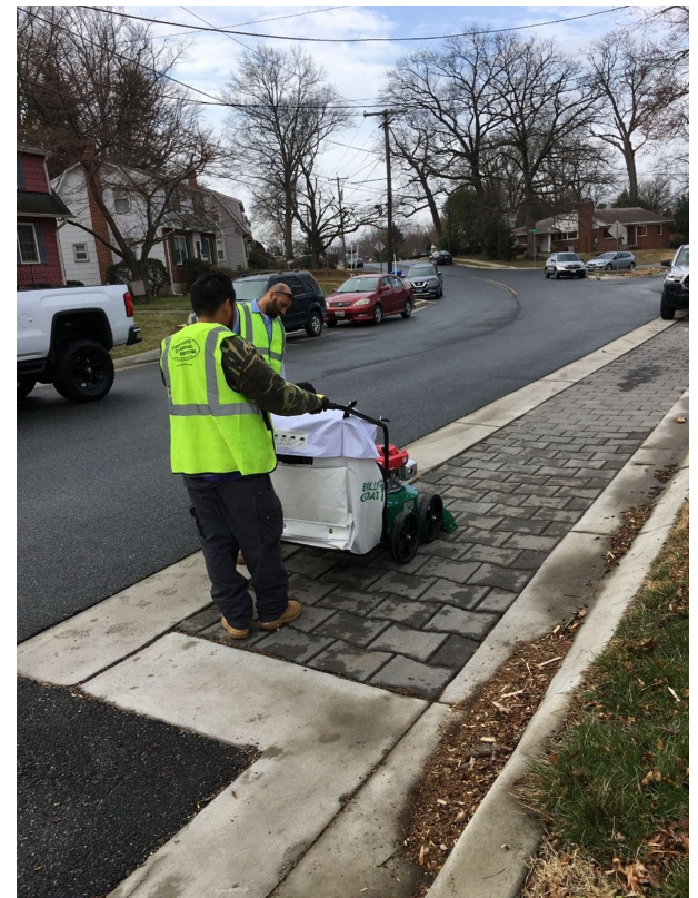
Pervious Pavement Cleaning
