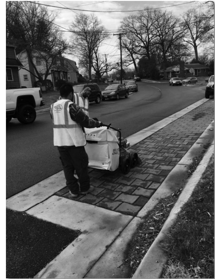
Pervious Pavement Cleaning
