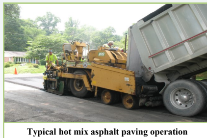
Typical hot mix asphalt paving operation
