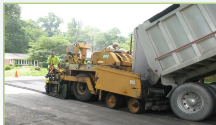
Typical hot mix asphalt paving operation
