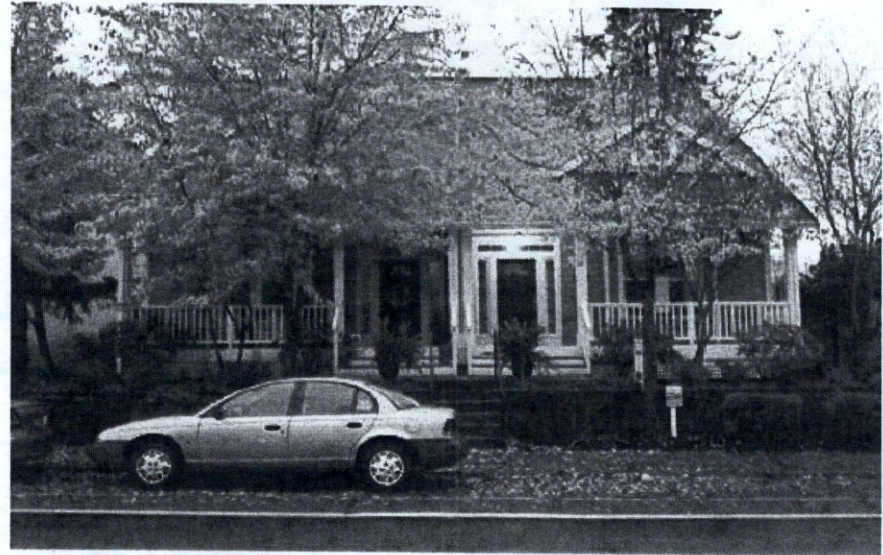
New Infill Duplex, Olympia, WA Credit: Olympia City Council
