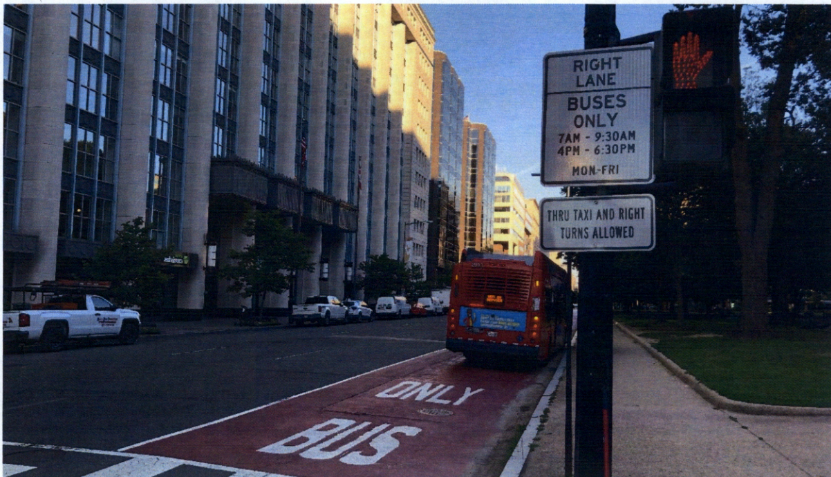
Curb Lane Transitway in Washington, DC
