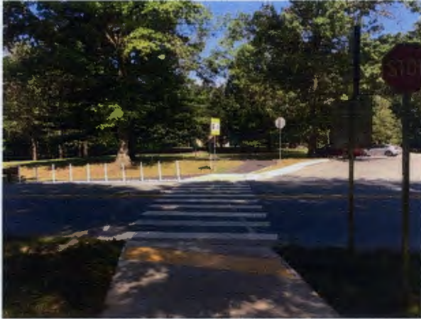
Garrett Park Road crossing of the Rock Creek Trail. Improvements included:
