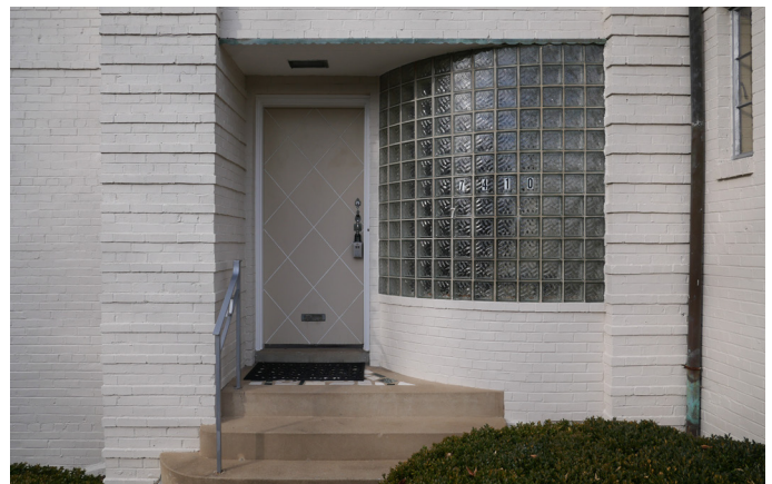
Figure 11: View of the front (east) elevation, 2020. The façade features a sweeping curved glass block wall that leads to the recessed main door. Source: Historic Preservation Program.
