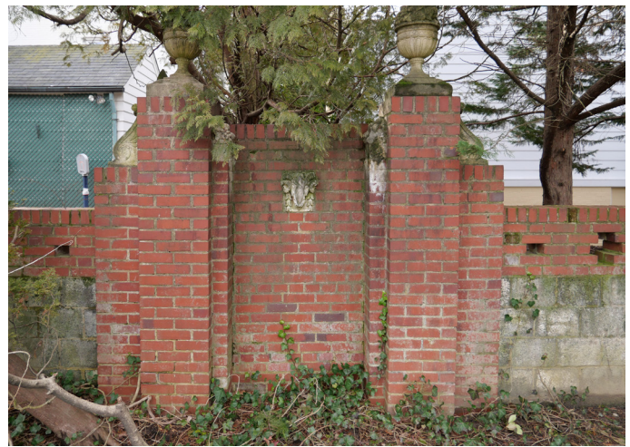
Figure 12: Detailed view of the brick and concrete block retaining wall. Source: Historic Preservation Program.
