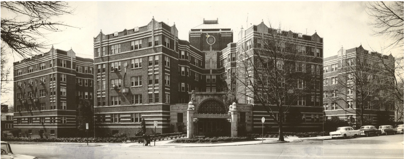
Figure 7: Mesrobian designed Sedgwick Gardens (Washington, D.C.) in the Art Deco style for developer Max Gorin in 1931. The apartment building is listed in the National Register of Historic Places.
